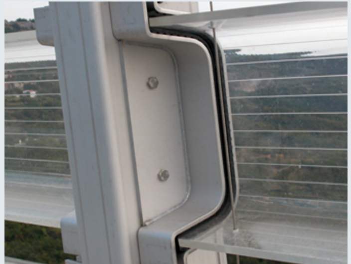
ACRYLITE® Soundstop Wind Barrier "C" shape design
