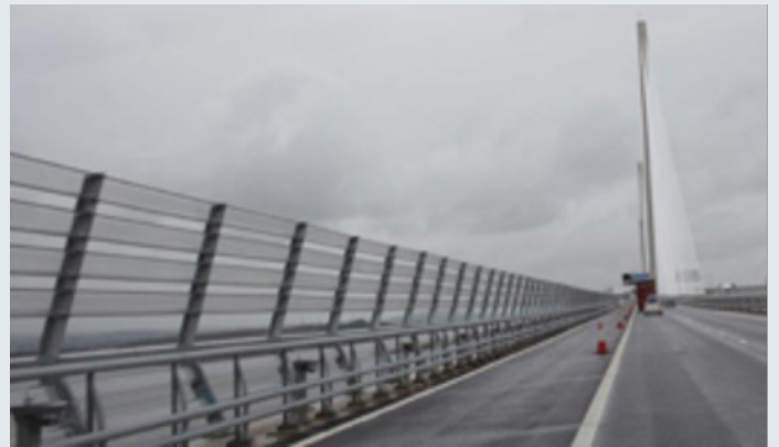
ACRYLITE® Soundstop Wind Barrier System with "C" shapes on the Queensferry Crossing Bridge in Scotland, UK
