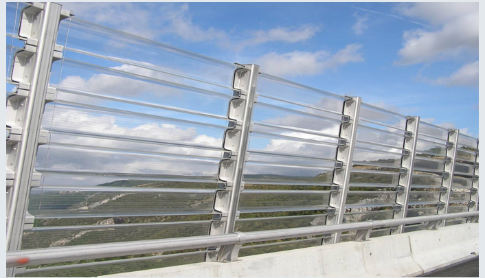
ACRYLITE® Soundstop Wind Barrier System with "C" shapes on the Crni Kal viaduct in Slovenia
