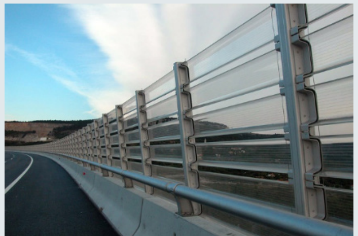
ACRYLITE® Soundstop Wind Barrier System with "C" shape design using colorless Soundstop GS CC on the Crni Kal viaduct in Slovenia
