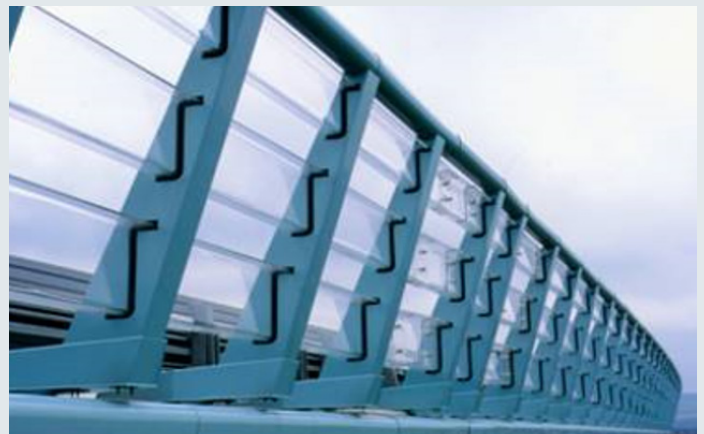
ACRYLITE® Soundstop Wind Barrier System with "Z" shapes on the Echingen Viaduct Boulogne-Sur-Mer In France
