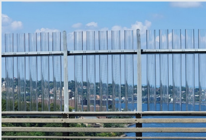
ACRYLITE® Soundstop Wind Barrier System with “C” shapes on the Verrazano Bridge in New York City
