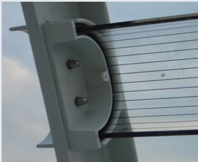
ACRYLITE® Soundstop Wind Barrier "Half Pipe" design
