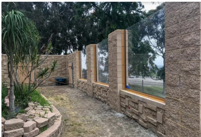
ACRYLITE® Soundstop Masonry Wall Type IA panel in Chula Vista, CA
