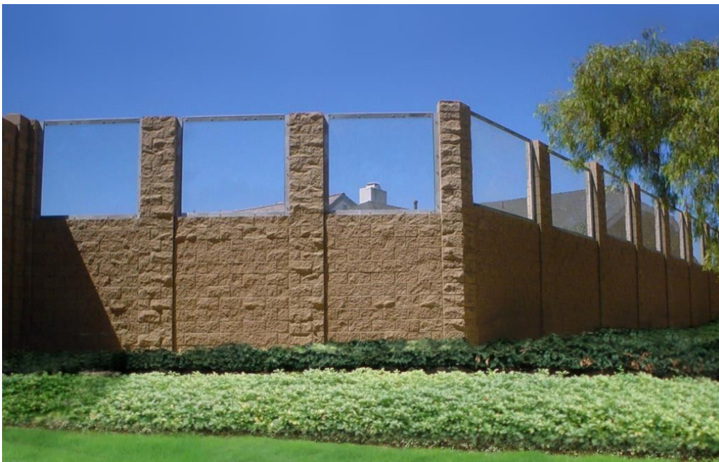
ACRYLITE® Soundstop Masonry Wall Type IB panel in Laguna Hills, CA
