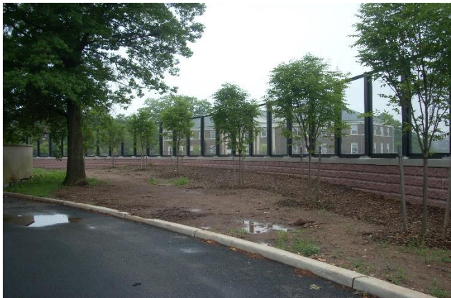
ACRYLITE® Soundstop Ready Fit System with black powder coated aluminum frames on Route 18 in New Brunswick, NJ
