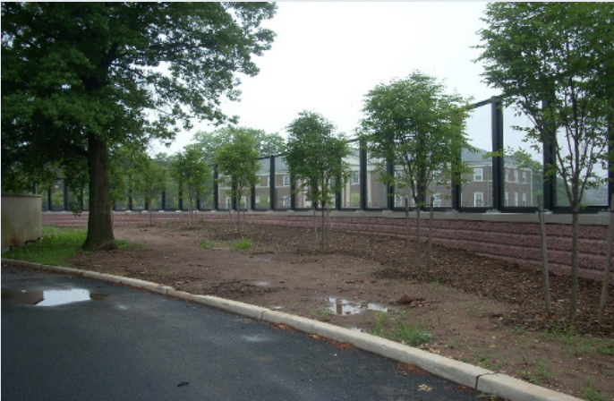
ACRYLITE® Soundstop Ready Fit System with black powder coated aluminum frames on Route 18 in New Brunswick, NJ
