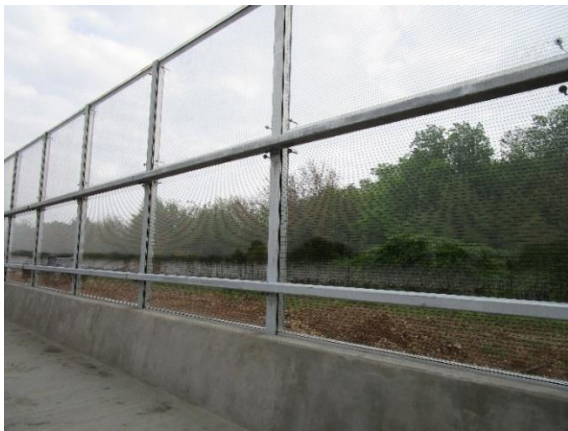
Example installation of a TL-4 System
